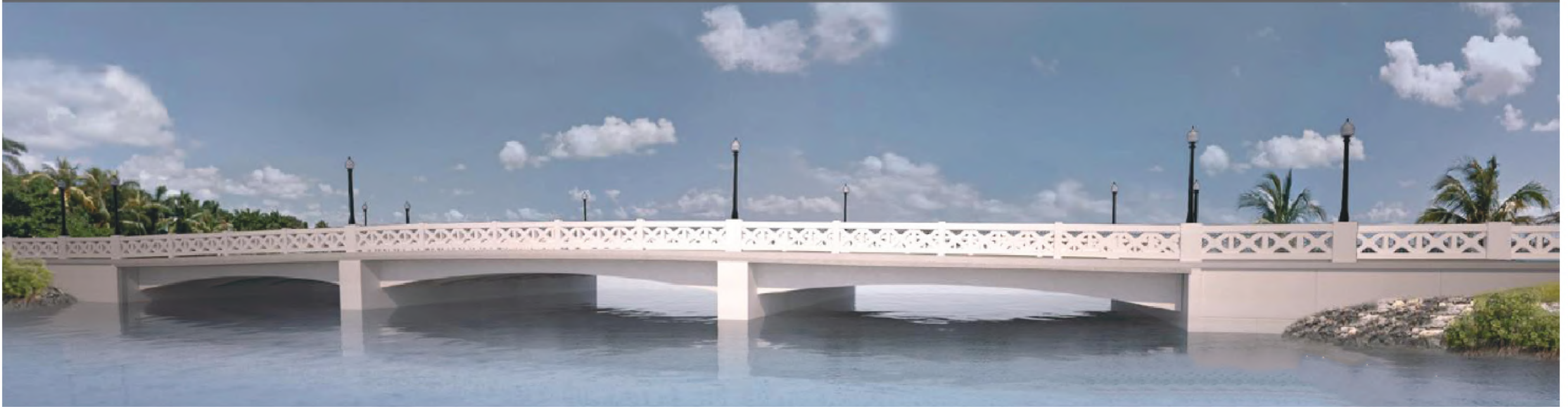
Fixed Bridge Alternative 7 – Arched Beams
